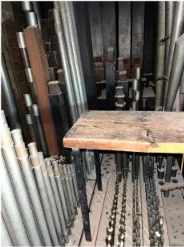
Pipework of the Great division
